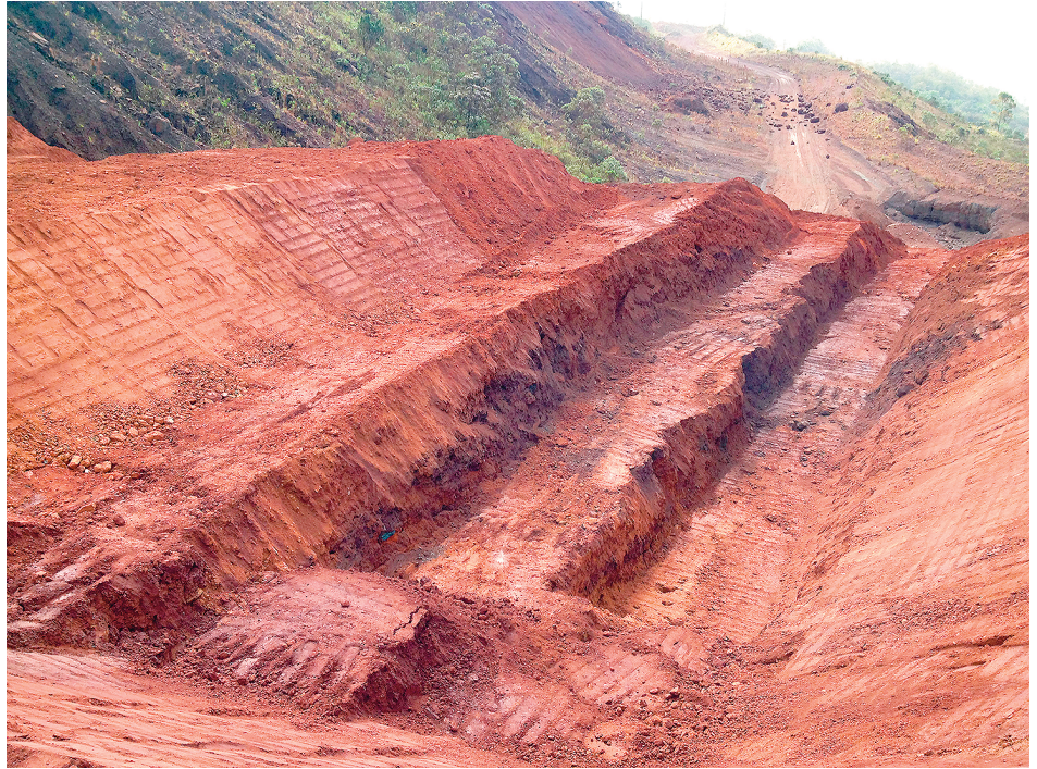
Figure 3 One-meter high berms modeled for testing in the bench dump.
